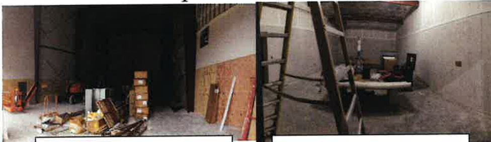
Apparatus Repair Bays
