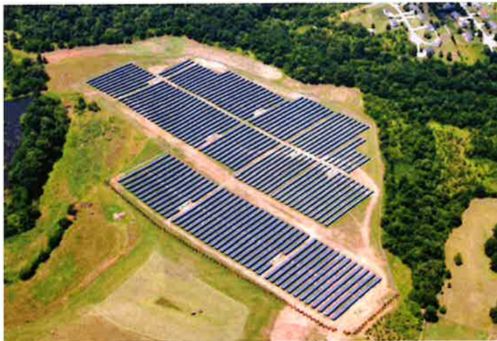
Figure 1: Utility-scale solar facility (5 MW AC ) located in Catawba County. Source: Strata Solar
